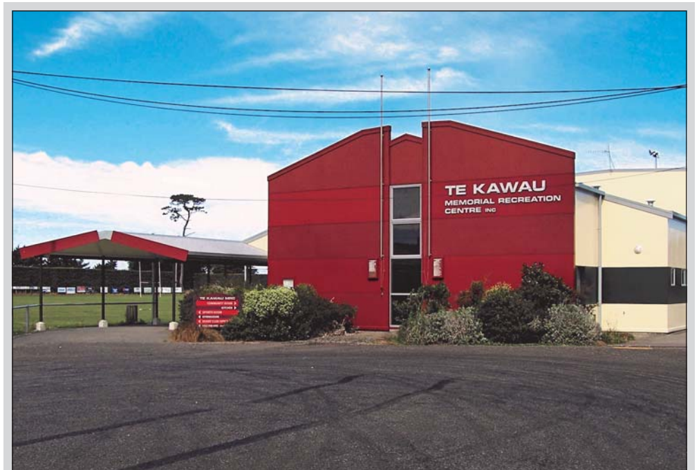
CONTRACTORS have recently completed an exterior repaint of the Te Kawau Memorial Recreation Centre at Rongotea. Painter Paul Manley said it was the building's first repaint since its construction about 10 years ago and settled weather had allowed them to complete the job in three weeks. Apiti's Community Hall, memorial archway and public toilet block have also benefited from a recent spruce-up.
