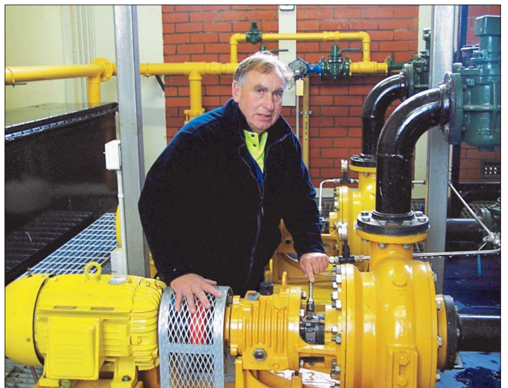
SUPERVISOR Russell Dean checks out a sludge pump in the digester building at the Wastewater Treatment Plant in Kawakawa Road, Feilding - his workplace for the past 35 years.
