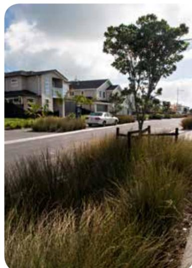
Planted Swales and open drains to manage stormwater on a localised level
