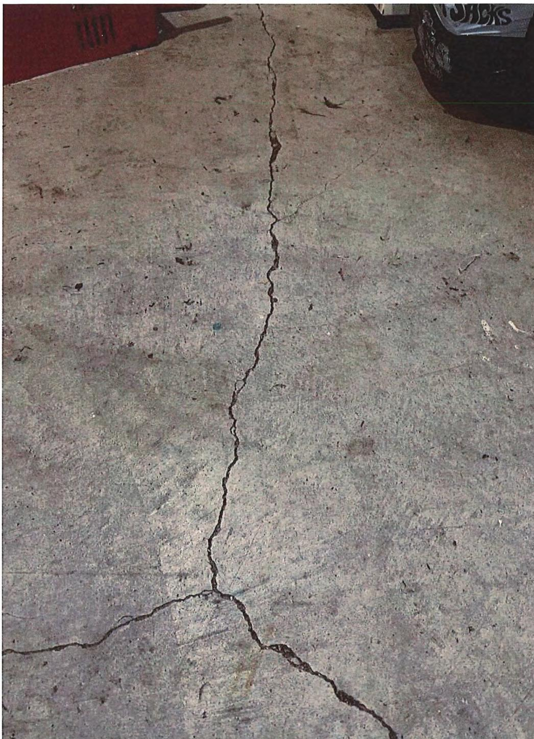
***Photo 5: View of concrete floor inside the garage shown on photos 1-3 showing existing damage to the concrete floor from the root system of Tree 6***
