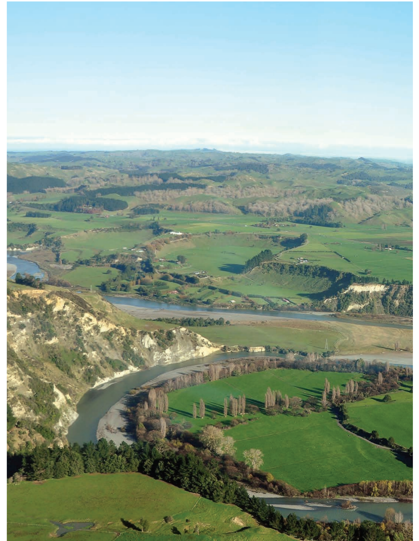
Rangitikei Photo 3- High voltage Bunnythorpe to Ongarue A (110Kv) transmission line crossing the Rangitikei River
