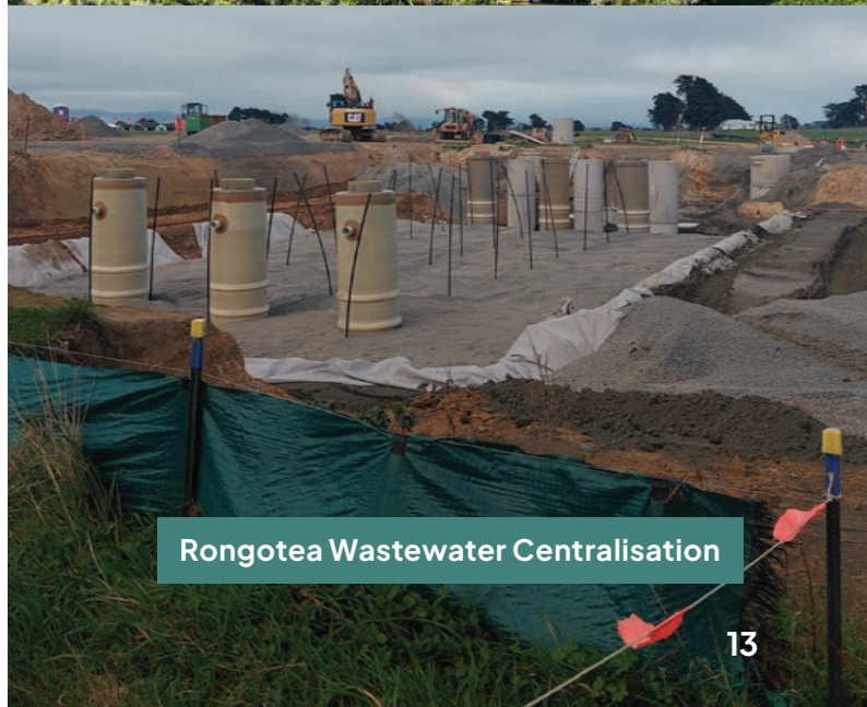
Rongotea Wastewater Centralisation
